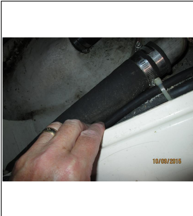
Cracked exhaust hose.
