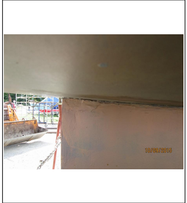
Gap between keel and hull.
